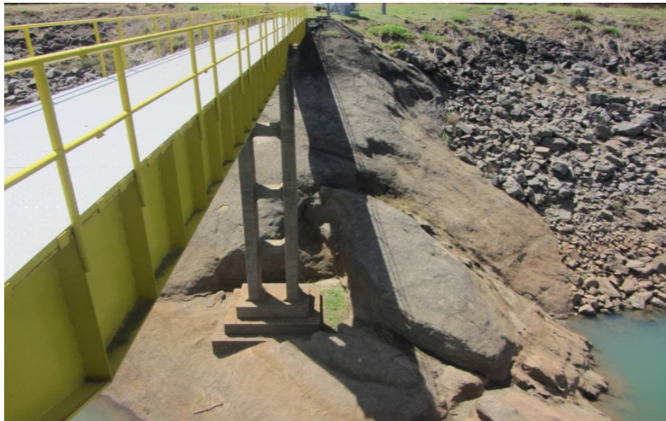
FIGURE 11: View from the footbridge, supported on concrete columns and foundation blocks.
