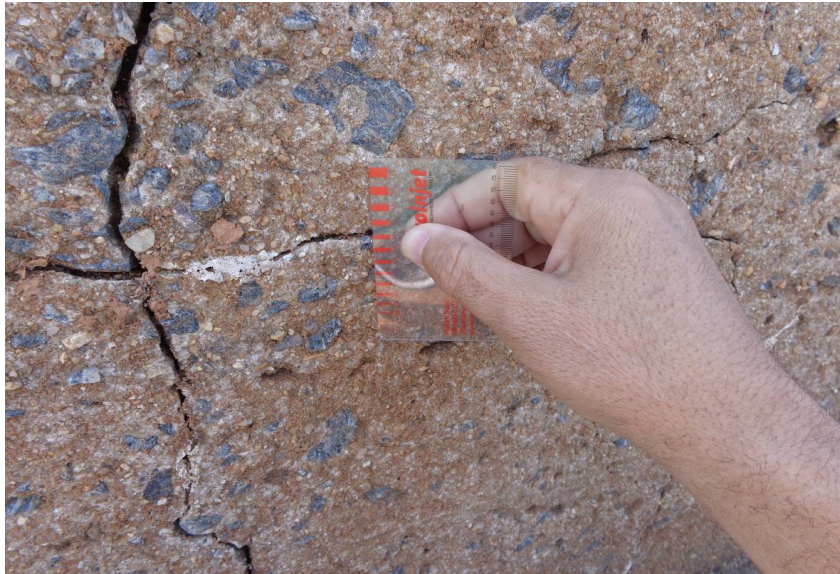
FIGURE 15: Detailed view of the Foundation blocks, measuring the opening of cracks on the order of 2.0 mm. Observe the resulting gel of the AAR.
