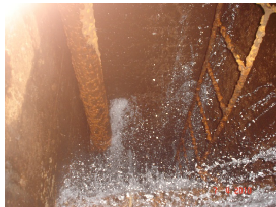
FIGURE 4 FIGURES 4 and 5: Infiltration through cracks of wall ventilation tunnel.
