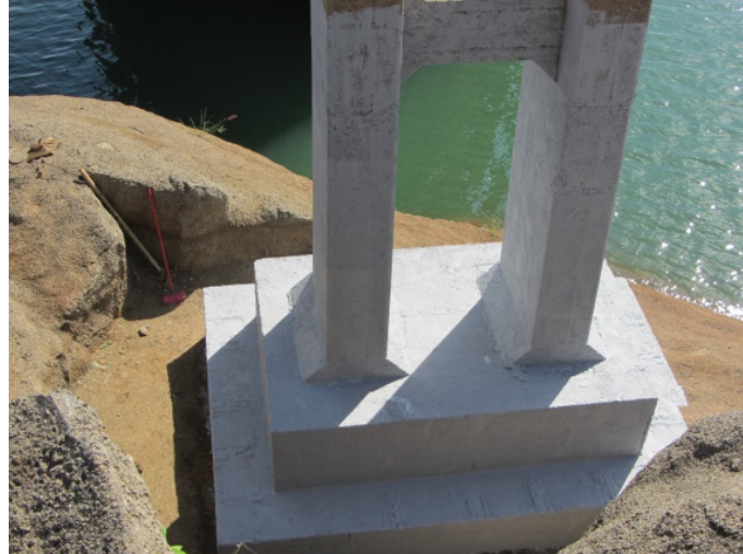
FIGURE 18: View from the set blocks and concrete columns, texture coating, after the injection job.
