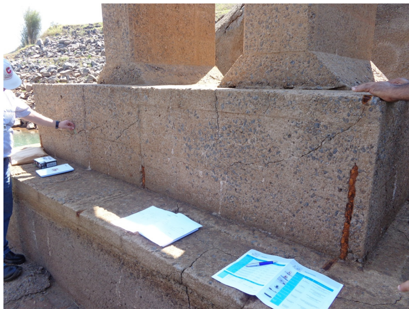
FIGURE 14: View from the block of the concrete columns, highlighting the cracks, with top opening up to 1.0 mm. Presence of leaching and segregation on the concrete surface.
