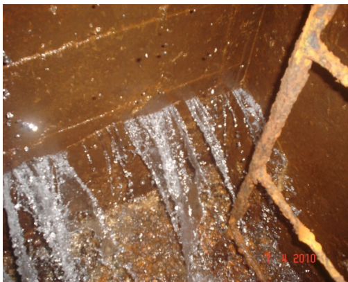
FIGURE 4 FIGURES 4 and 5: Infiltration through cracks of wall ventilation tunnel.
