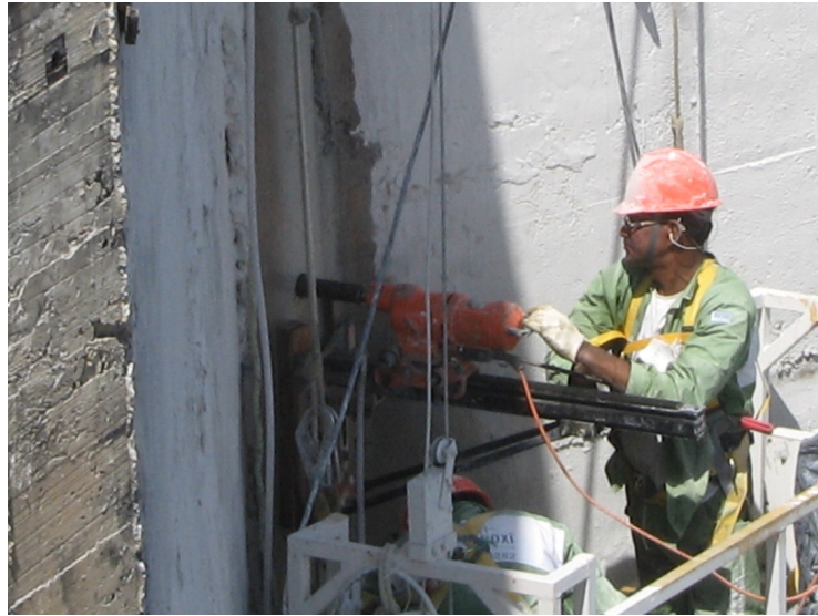
FIGURE 7: Relief hole horizontal drilling.
