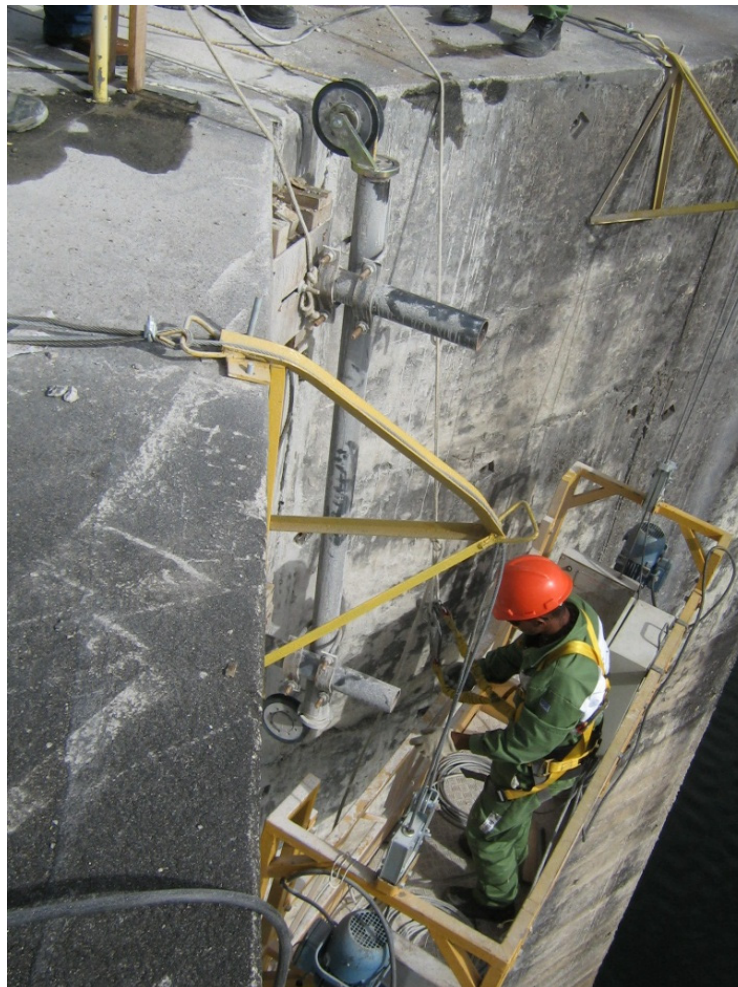
FIGURE 8: Cable guiding system and suspended working platform.
