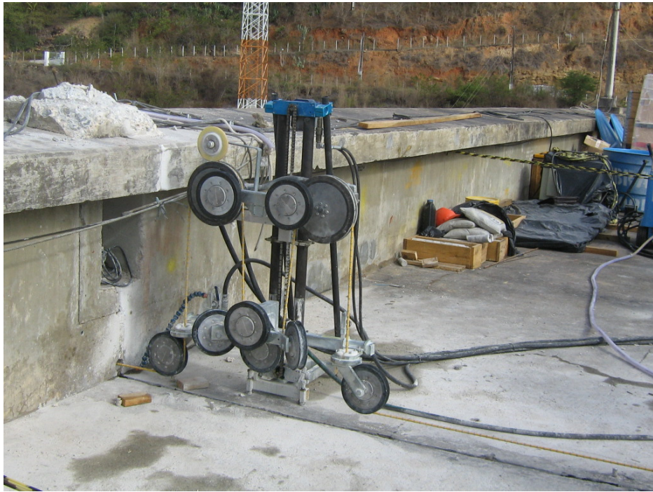
FIGURE 5: Cutting equipment at dam crest near downstream parapet wall.
