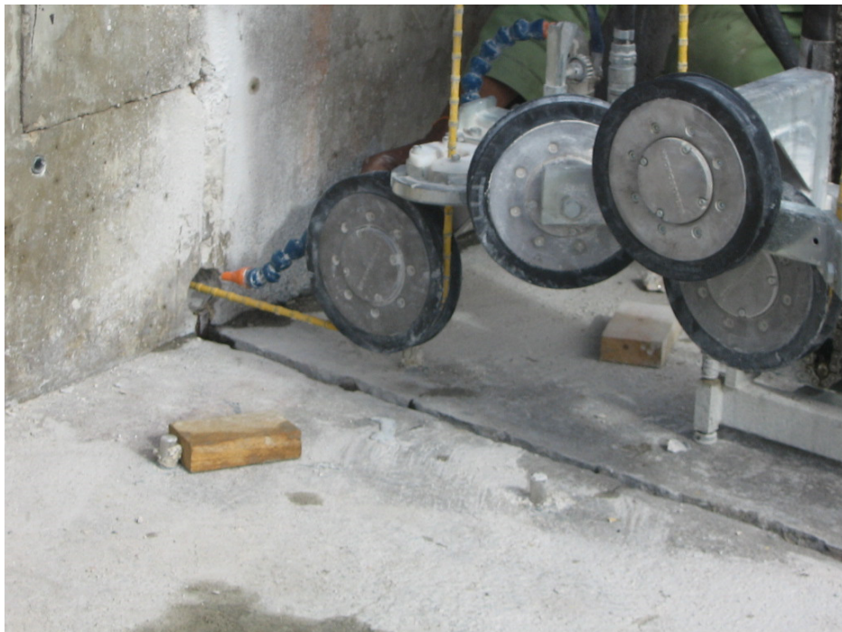
FIGURE 6: Detail of diamond coated cable and water cooling system.
