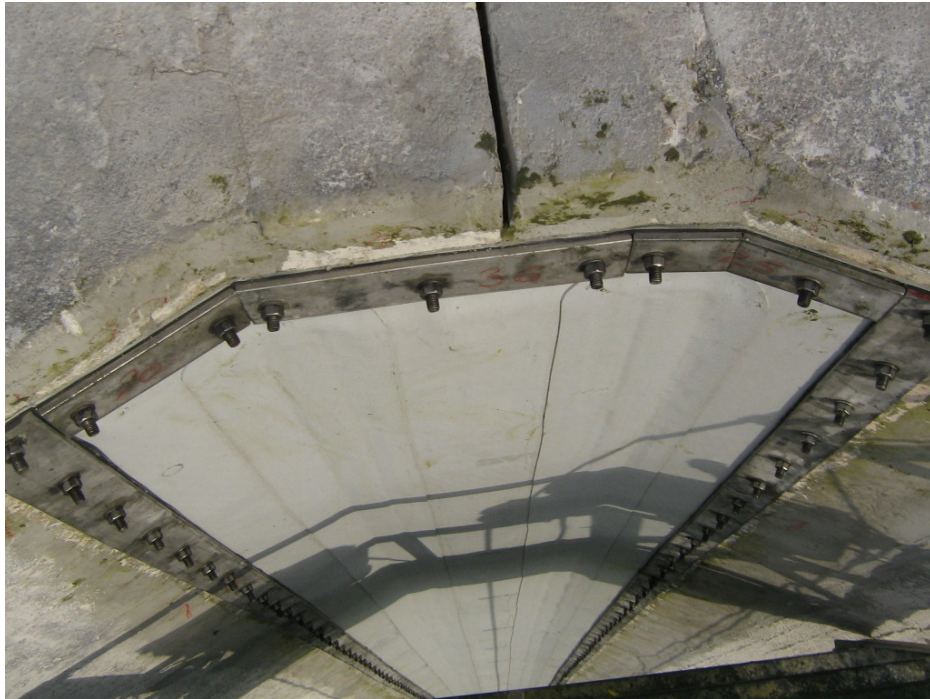
FIGURE 9: Slot and geomembrane sealing system after completion.
