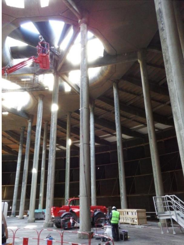
FIGURE 5: A view of some of the pillars and the concrete slab with one of the fans.
