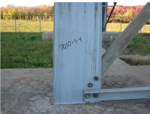
FIGURE 9: Example of a foundation with a greywacke aggregate (2013 inspection).
