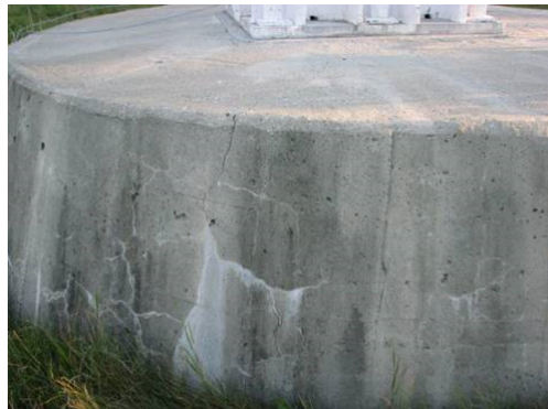
FIGURE 8: Example of an encapsulated foundation repaired in 1996 (2013 inspection).
