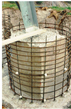
FIGURE 15: Steel reinforcement in place (1986-1987 works).
