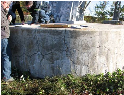
FIGURE 5: Example of a foundation injected in 2001 (2013 inspection).
