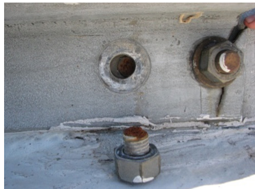
FIGURE 10: Example of ruptured bolt and steel angle (2013 inspection).
