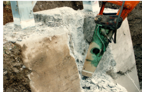
FIGURE 14: Example of a foundation under partial splitting (1986-1987 works).
