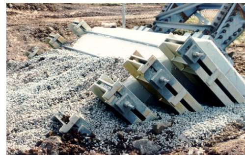
FIGURE 18: Example of a membrane and a post-tension frame (1986-1987 works).
