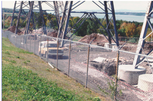
FIGURE 13: Example of repair works done in 1986-87 (splitting and encapsulation).
