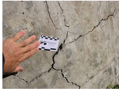
FIGURE 6: Close-up of wide cracks (2015 inspection).
