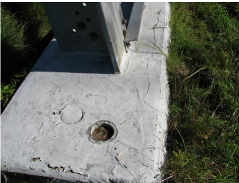
FIGURE 7: Example of a foundation covered with a membrane (2013 inspection).
