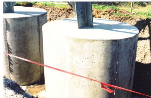
FIGURE 16: Encapsulation with new concrete (1986-1987 works).
