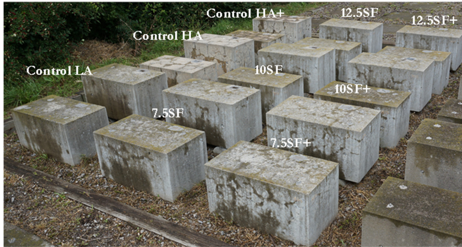
Figure 8: Exposure blocks incorporating the moderately-reactive Su aggregate. Each mix is represented by two blocks, one sitting directly on the ground and the second one sitting on small concrete supports so the block stands above ground. The mixtures correspond to low-alkali and high-alkali (unboosted and boosted) controls, and unboosted and boosted (“+ series”) specimens incorporating 7.5, 10% and 12.5 silica fume. The alkali content of the silica fume concrete mixtures can be found in the legend of Figure 10).
