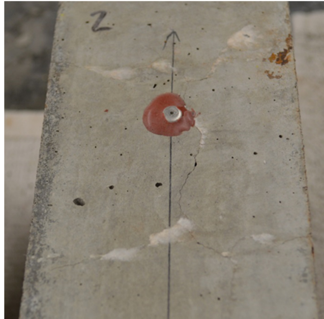
FIGURE 7: Cracking and efflorescence on a matching prism.
