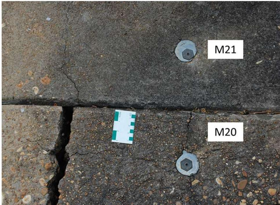
FIGURE 3: Monoliths 20 and 21. Crack openings in monolith 20 exceeded 25 mm in some locations.
