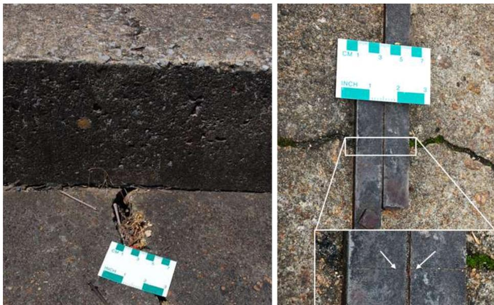
FIGURE 4: Overlay placement installed after decommissioning with no reflective cracking (left) and notched metal strips indicating no crack growth after installation (right).
