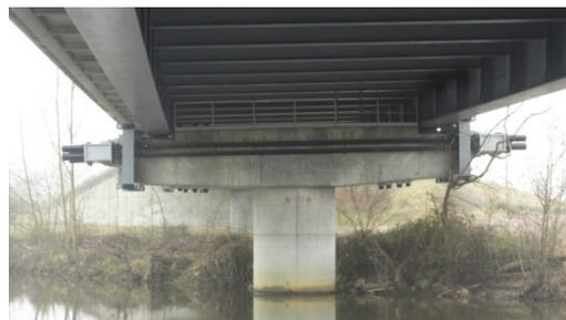
FIGURE 2: View of the Pier P1 with the cap beam strengthened by prestressing tendons.
