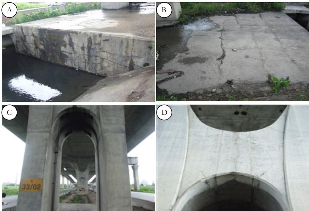
FIGURE 2: Overview of ASR-deteriorated structures. A, B: Pile cap (footing). C, D: X-type PC pier.
