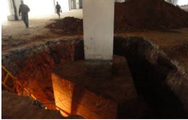
FIGURE 1: Edificio 10's pile cap.
