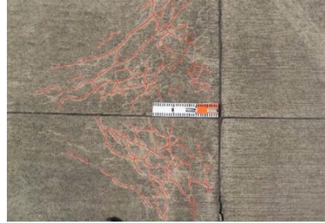
FIGURE 2: Cracks on the corner of pavement slab
