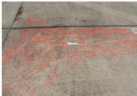
FIGURE 3: Cracks propagated along the slab joint
