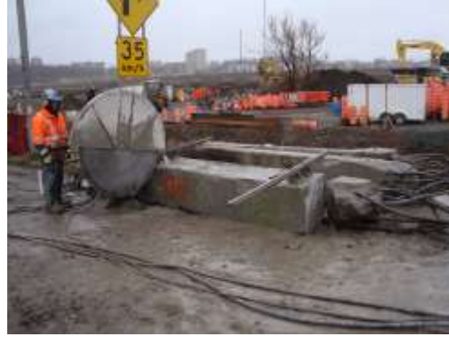
B - Sawing and preparation of the columns
