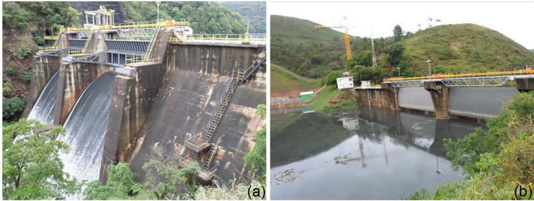
FIGURE 1: Downstream side (a) and upstream side (b) of Pirapora Dam.
