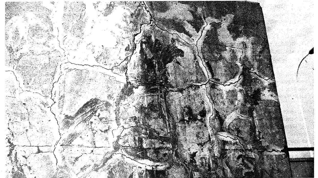
Figure 1 (a) Extensive cracking of exposed bridge portal. Attempts to seal the cracks by means of epoxy resin have failed.
