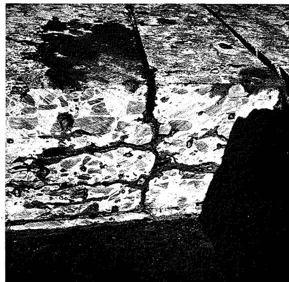
FIGURE 4: Evidence of vertical and horizontal cracking at a transverse joint.
