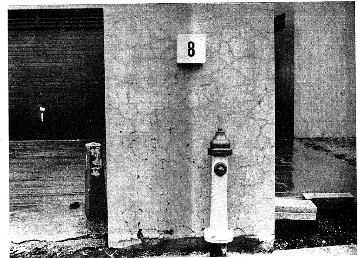
FIGURE 2: Most houses in Reykjavik, Iceland, are built of solid concrete. Changing building habits during the late '60s have caused alkali-silica hydration to become a cause of intensive cracking. The consequent repairs and added depreciation costs are more unpleasant for the individual, who puts his life savings into a house than for public bodies or industry which own plant and buildings which continuously form part of the earnings for depreciation.
