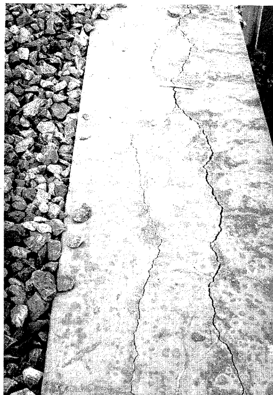
Fig. 4 - ASR distressed Abutment of a railway bridge (Equatorial Africa) :
