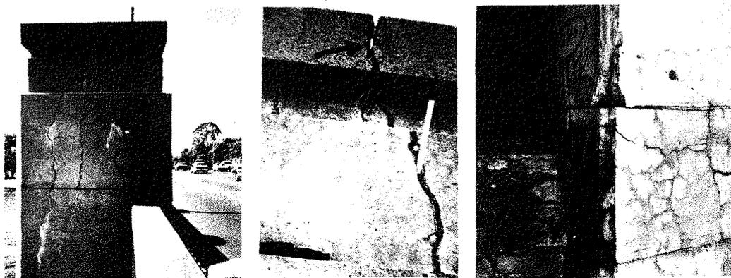
*Fig. 1.* Some features of cracking in various parts of the bridge, observed in 1992. Left and middle pictures show cracking in the top of a pylon, where some parts of the concrete have become separated (arrow). The right picture shows map cracking in the ground section of the pylon with some spalling.
