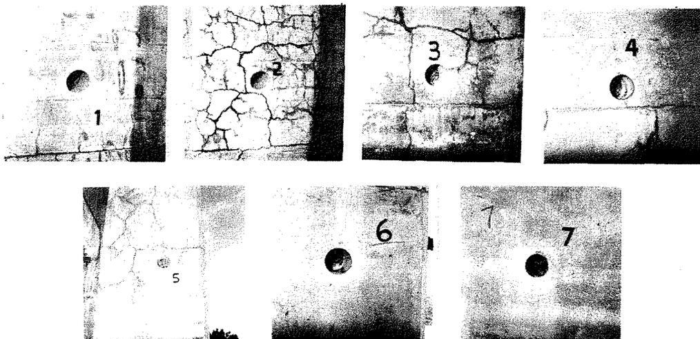
**Fig. 2.** Condition of concrete in various zones where cores were taken. Cores 1 - 5 came from the east abutment pier and columns, and cores 6, 7 from the west abutment columns.
