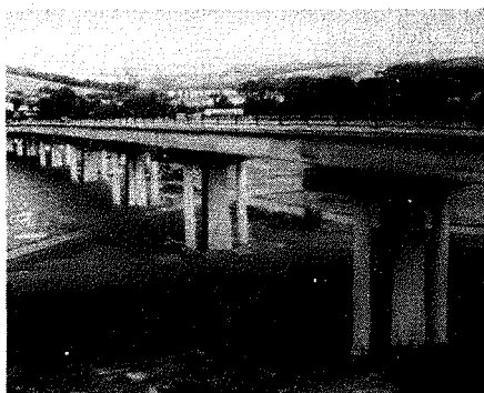
Figure 1. Marsh Mills Viaduct
