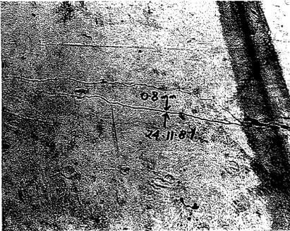
Fig. 5 Cracking in exterior beam
