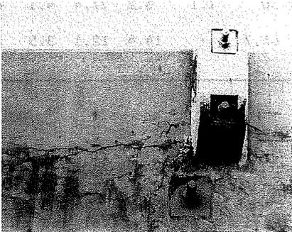
Fig. 3 Cracking in exterior beam
