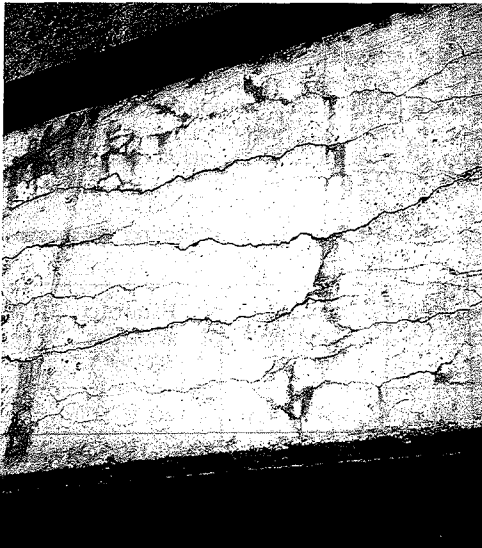
Figure 3. Cracking in a reinforced concrete beam.
