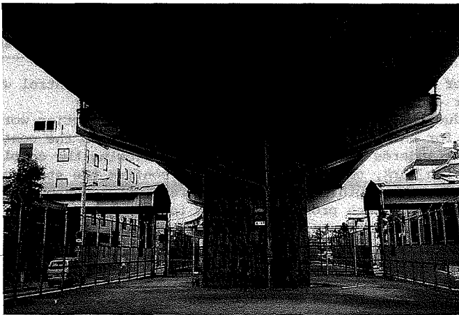
Photograph Repaired Concrete Structure
