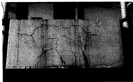
Figure 17 Beam repaired by epoxy resin
