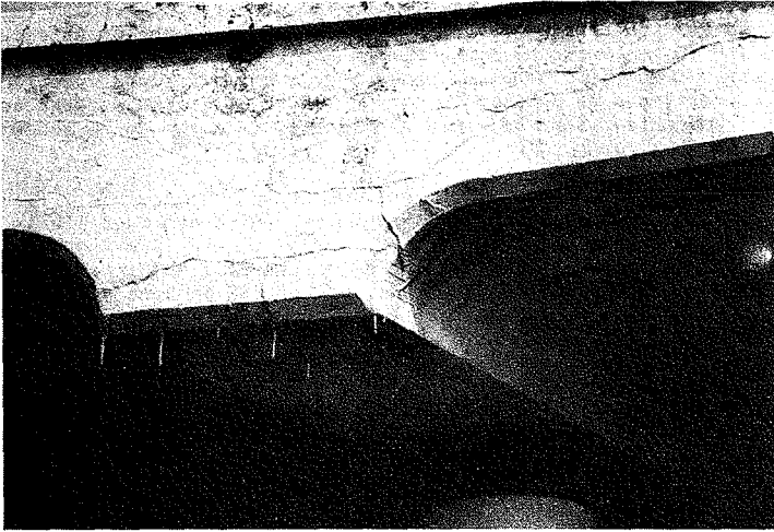
Figure 1 Cracks in the side of the road deck near a row of columns
