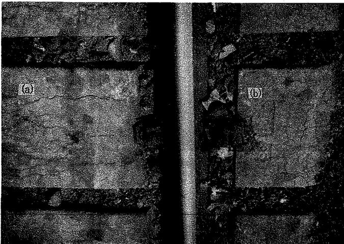
Fig. 2 Cracking of prestressed concrete railway tie (a) center, (b) end
