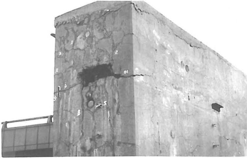
Fig. 2: Deterioration of concrete in portal as result of AAR
