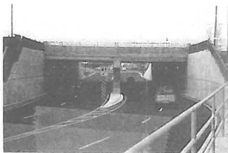
Fig. 9: Rehabilitated structure, November 1998. The replaced Elgin Street deck slab is in the foreground.
