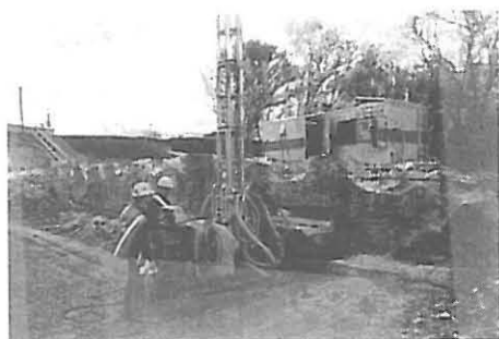
Figure 3: Removal of concrete by hydrodemolition
