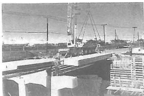
Fig. 8: Installation of precast concrete deck units, Elgin Street Overpass. The CPR structure is in the background.
