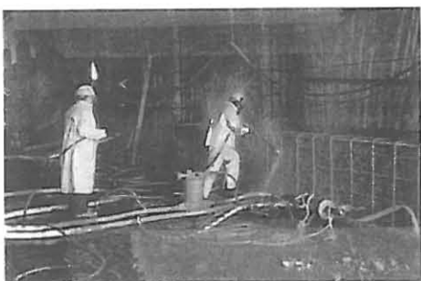
Fig. 4: Water blasting clean up and surface preparation of the roadway crash wall and piers prior to concrete refacement. Typically the outer 75 mm to 100 mm of deteriorated concrete has been removed and some steel reinforcement has been replaced.
