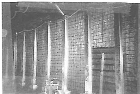
Figure 2: Commencement of formwork erection to the CPR structure abutment. At this stage the outer 200 mm of deteriorated concrete has been removed and the epoxy coated steel reinforcement and mechanical anchors are in place. Note the temporary steel structure supporting the bridge deck beams under the CPR rail lines.
