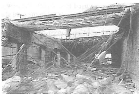
Fig. 7: Demolition of Elgin Street cast-in-place deck slab. The CPR structure is in the background.
