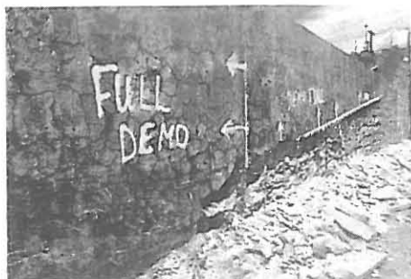
Figure 1: Severe AAR deterioration in structure retaining wall. Generally the outer face steel reinforcement is corroded.
