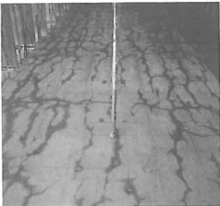
Fig. 5: ASR cracks occurred on the surface of the column
