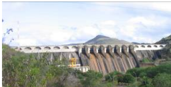
Figure 2: General downstream view of Pedra Dam.
