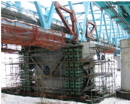
Figure 14: Supporting by temporary bent
