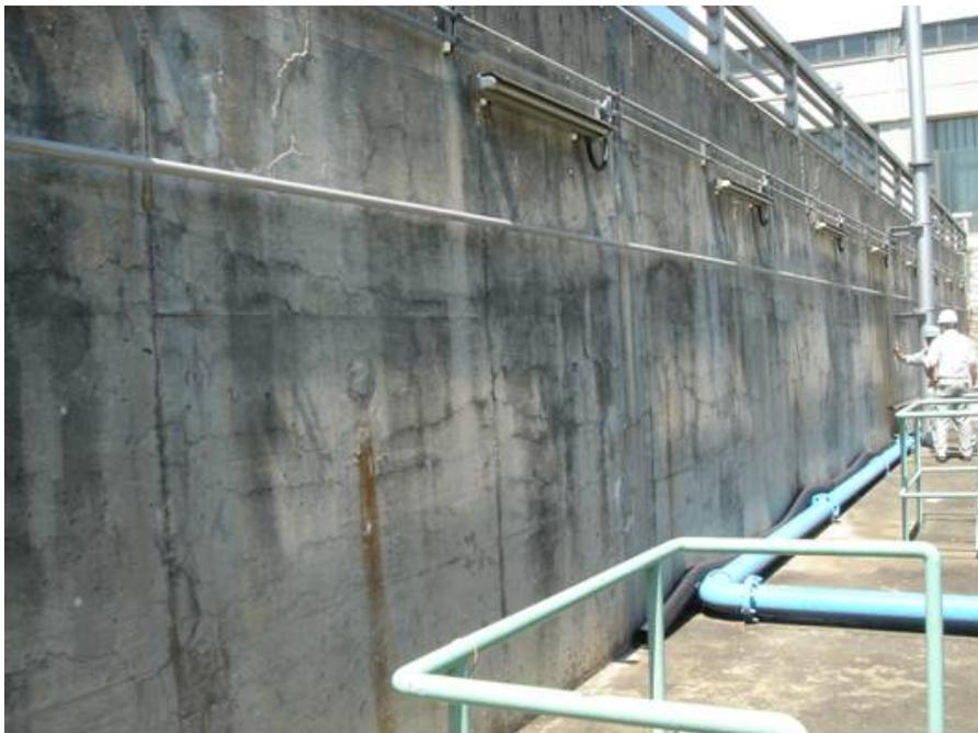
Figure 4: Retaining wall B (before injection)
