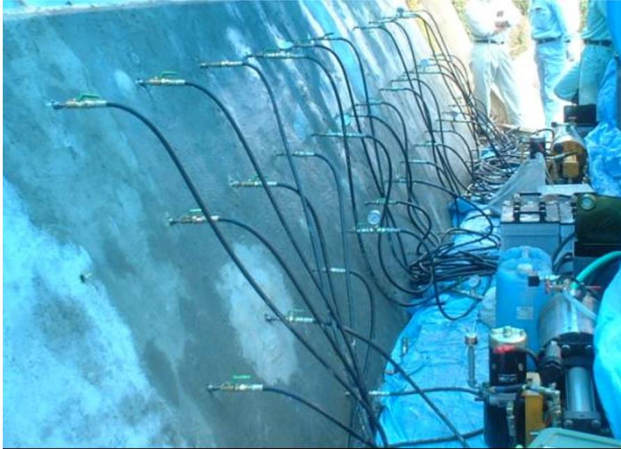
Figure 3: Retaining wall A (injection)
