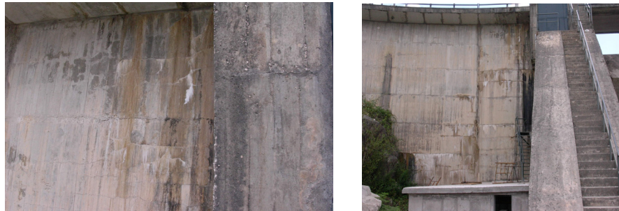
Figure 2: Horizontal cracks and map cracking in the right buttress and in the right arch.
