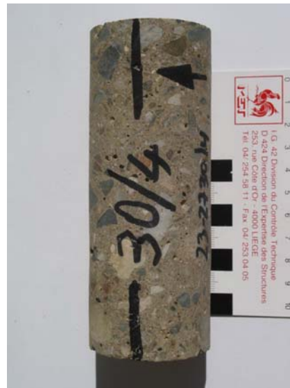
Figure 5: Bridge H after the “GCG-DUG” test. Concrete is still in good condition (ø 50 mm).
