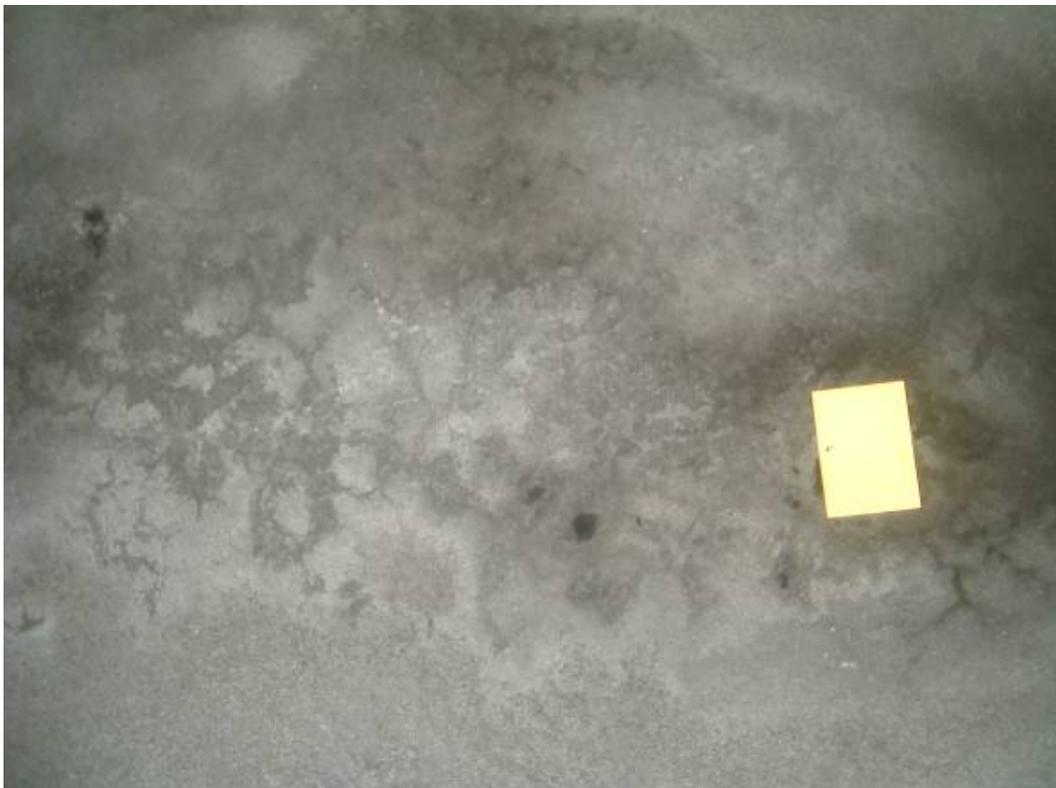
Figure 1: AAR suspect area with surface cracks. Core was taken for further examination. The card is 75×105mm, and shows the location of the core.
