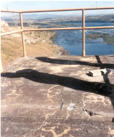
Figure 2a: Crack along transversal section of a spillway column
