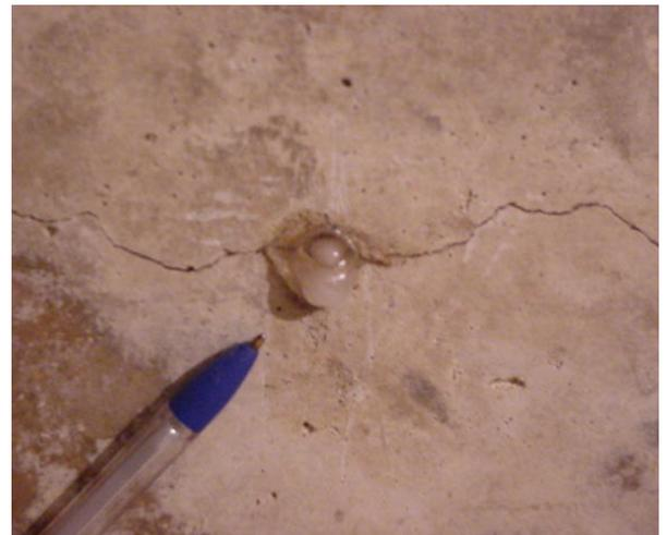
Figure 2b: ASR Gel from cracking in the concrete surface of the spillway driftway.
