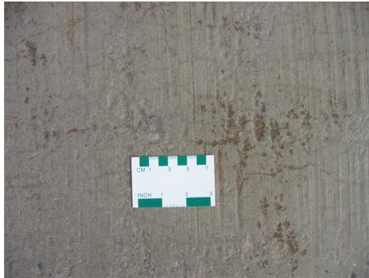
Figure 1: Fine map cracking on 100% PC concrete slab in 2004 at 6 years.
