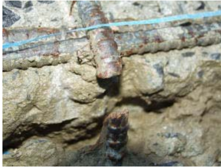
Figure 1: Fractured stirrup
