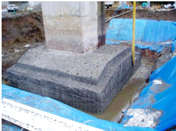
Figure 11: Footing after chipping away concrete.
