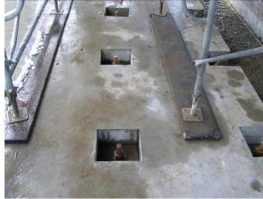
Figure 14: Layout of vertical prestressing steel bar.
