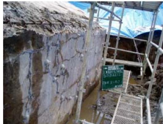
Figure 5: Enlarged view of deteriorated concrete at the edge and sides of the footing top.
