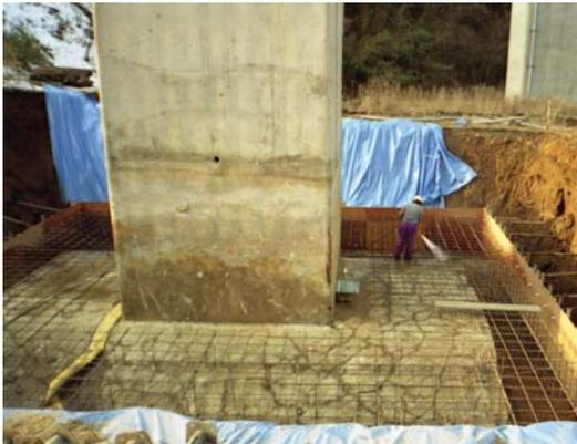
Figure 4: Deteriorated concrete at the footing top.
