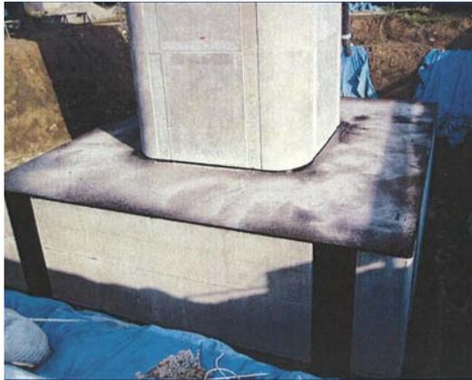
Figure 15: Bridge pier after the strengthening.
