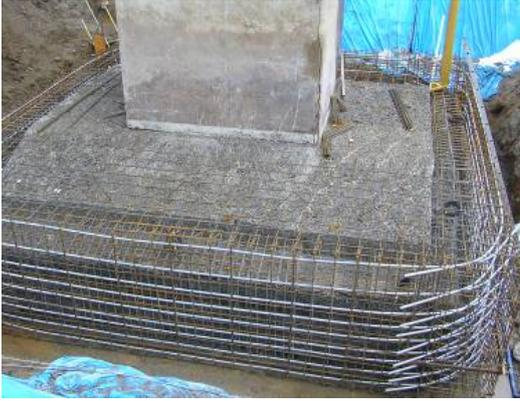
Figure 13: Layout of prestressing steel strand around periphery of footing.
