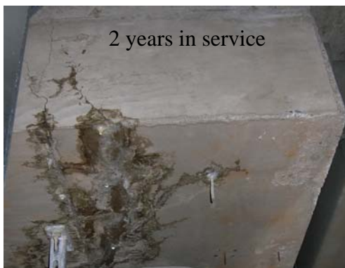
Figure 2: Visually evaluated increase in water leakage through cracks in the water gutter. Photos taken in May 2006 (upper), November 2006 (left) and June 2007 (right).
