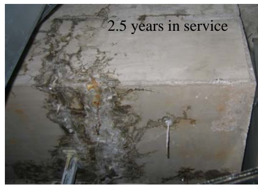
Figure 2: Visually evaluated increase in water leakage through cracks in the water gutter. Photos taken in May 2006 (upper), November 2006 (left) and June 2007 (right).
