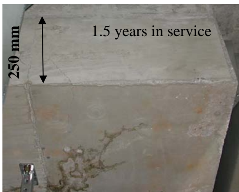
Figure 1: Map cracking on the outside face of the pool wall. Note that the cracks are intensified by drawings on the photo.
