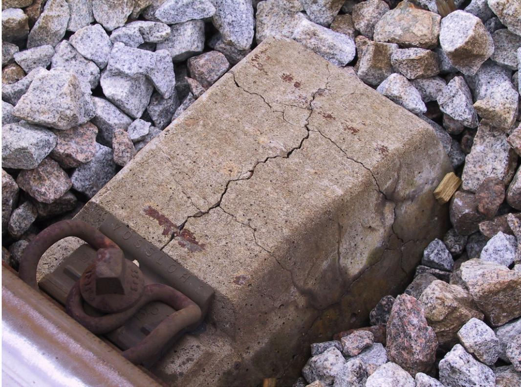
Figure 1 – End view of a cracked concrete railway sleeper.
