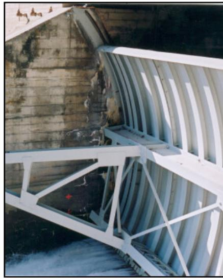
Figure 5: Radial gate wall of a dam in southern BC exhibiting ASR distress
