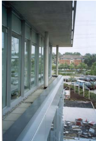
Plate 1: Columns and soffits of investigated office building, Hampshire.
