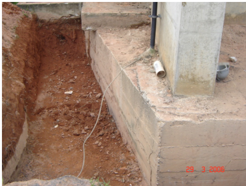
Figure 1: Start of excavation around the AAR-affected foundation block.
