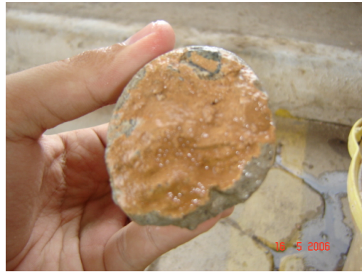
Figure 8: Removal of specimen before washing with the inner face of the crack soiled by clay material.
