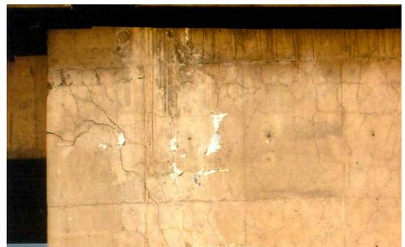
Figure 1: ASR map cracking on the bridges in the vicinity of Izmir
