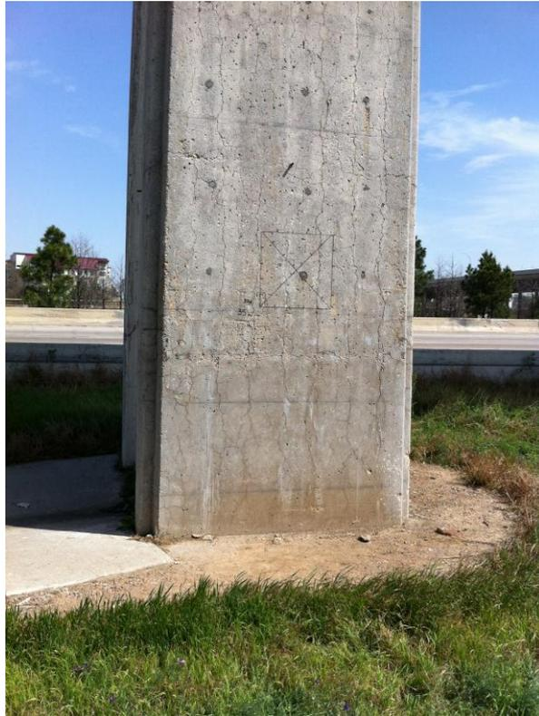
FIGURE 5: Etched surface from the electrochemical lithium migration column 46
