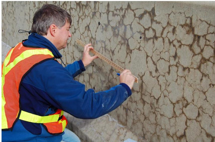
FIGURE 2: Photo of a typical Jersey barrier treated in Leominster, Massachusetts. A grid is being drawn on the surface of the barrier for the determination of the Crack Index [6].
