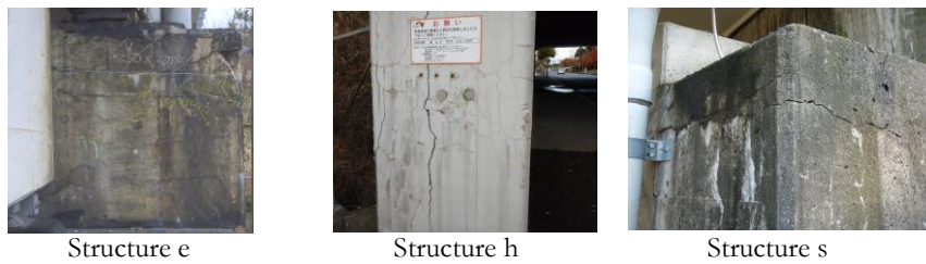
FIGURE 2: Deterioration due to ASR
