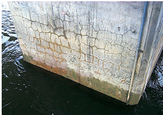
Figure 1: Typical crack pattern for DEF, very similar to AAR ones
