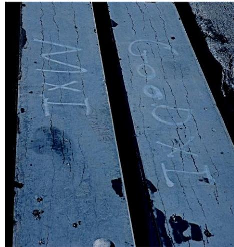
Figure 3- cracking in the soffit of planks M67 (left) and M12 (right) highlighted by wetting
