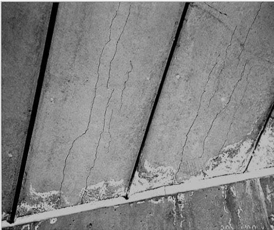
Figure 2- Longitudinal parallel cracking in the soffit of deck planks
