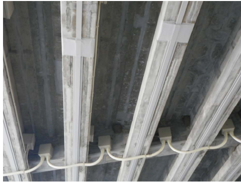
FIGURE 10: The repair of PC girders by cathodic protection method.
