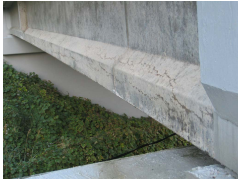
FIGURE 4: The cracking of T-shaped pre-PC girder (Rg).
