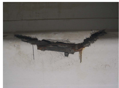
FIGURE 9: The CFRP sheet and girder broken.
