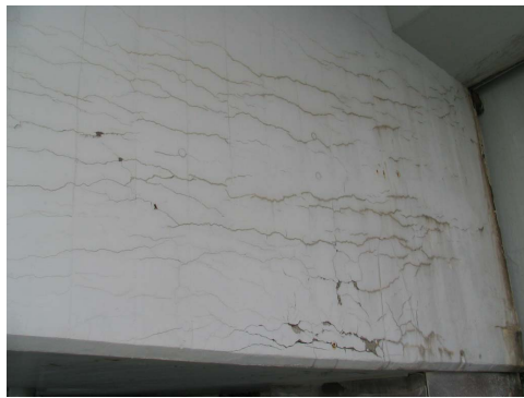
FIGURE 6: The cracking of hollow-core box type post-PC girder (Rg).
