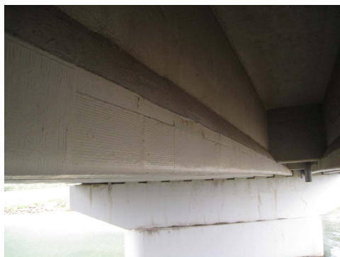
FIGURE 8: The strengthening of PC girders by CFRP sheet bonding method.
