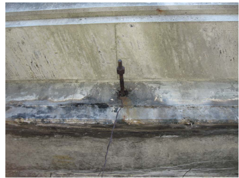
FIGURE 7: The transverse prestressing bar fractured.
