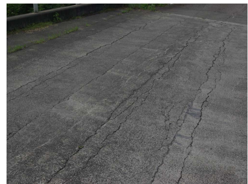
FIGURE 3: The reflection cracking on asphalt pavement.
