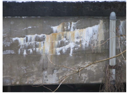
FIGURE 5: The cracking of hollow-core box type post-PC girder (As).
