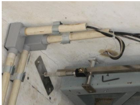
Figure 8: LVDT installed at the site
